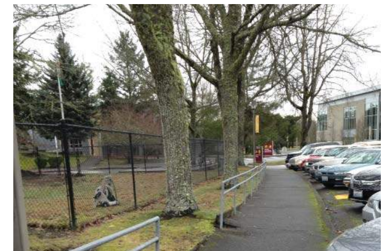
Trees planted too close to walkways can cause pavement damage. Root barrier or rigid foam under paving can be used in the future to avoid uplift. For existing uplift, asphalt can be removed and an air spade used to excavate around tree roots. Some roots can be cut and the area around the roots can be backfilled with graded base and the asphalt replaced with concrete.
