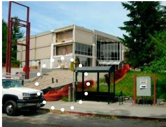
At Cascade Building, south entrance.
